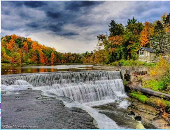
Beebe Dam Bridge
