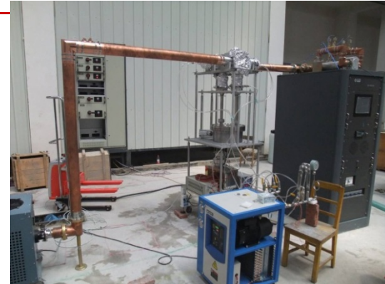
High power test stand
